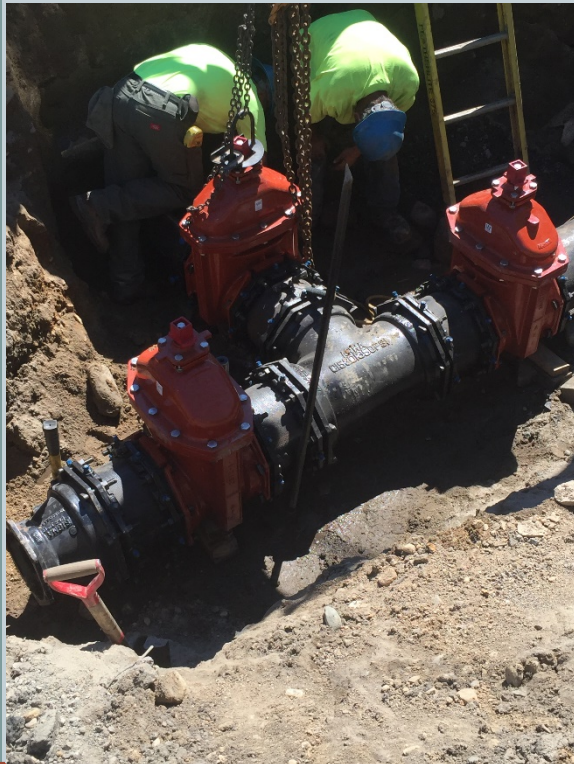
Installation of Tri-Valve at corner of North Main & Pascoag Main in 2016
