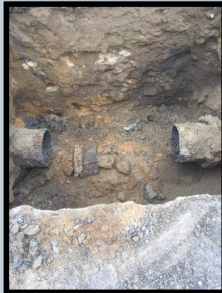
Cleaned and Lined and ready for reconnection
