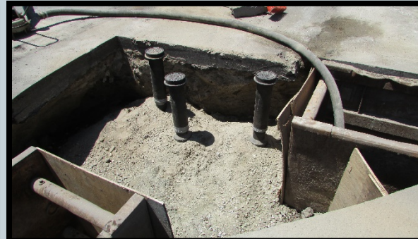
Tri-valve on Main/North Main intersection
