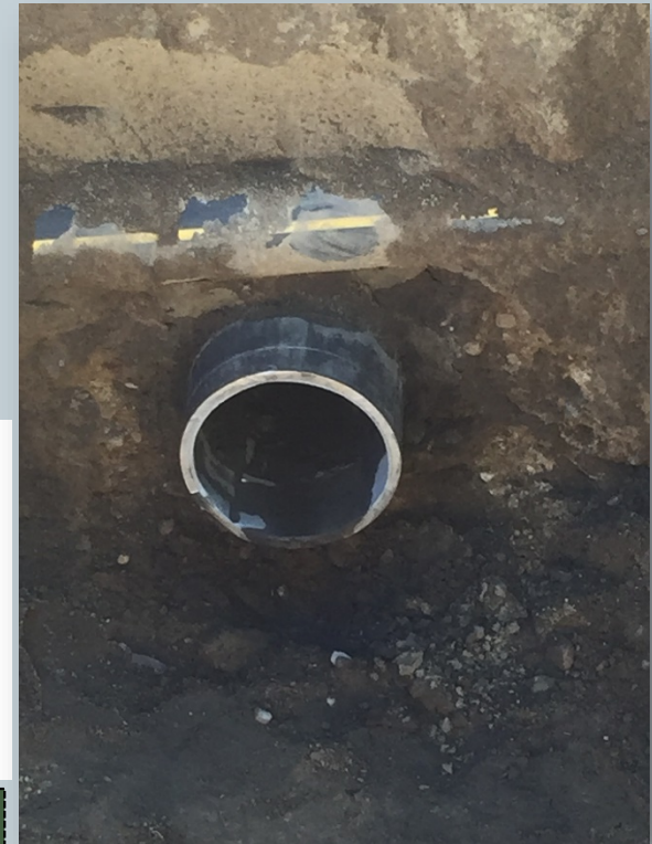
Section of water main after cleaning and lining, before reconnection
